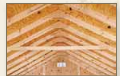
Collar ties are used on all buildings over 18' long.
